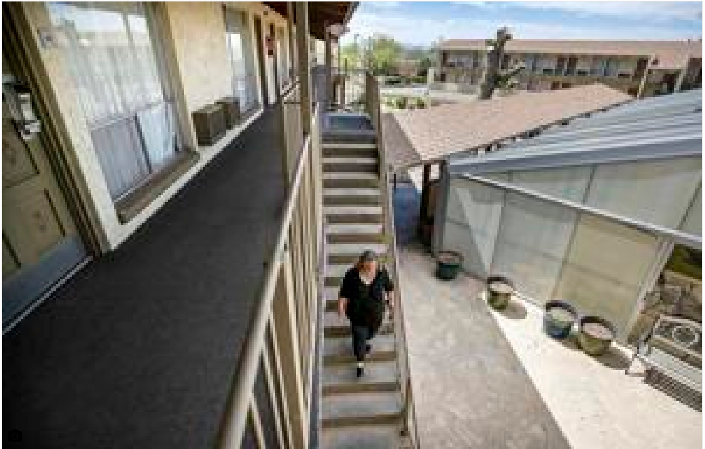
Conversion of Lamplighter Inn into affordable housing awaits design OK from Santa Fe
